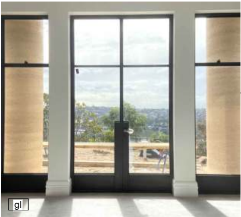
metal framed windows
