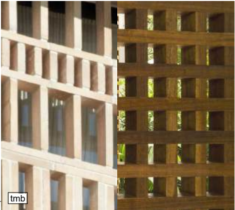
sliding timber shutters (to replicate brs pattern)
