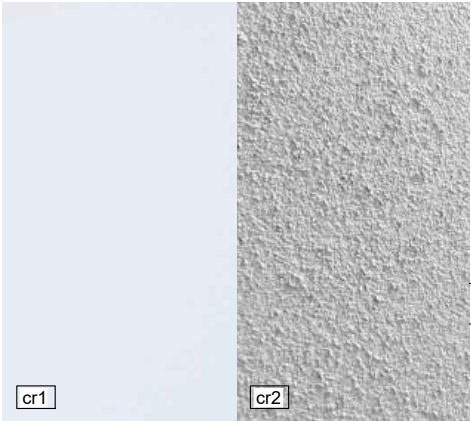
cement render roughcast cement render
