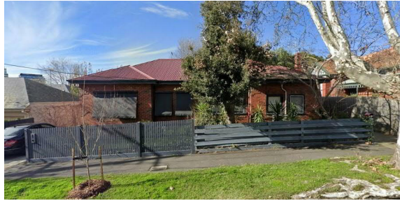
D - 1A & 1B HASTINGS ROAD - VIEW FROM WEST
